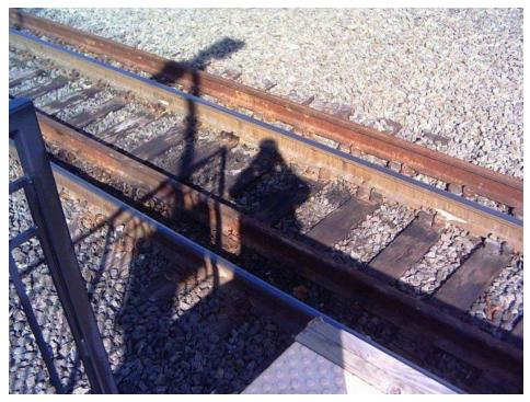
Figure 5-6. Gauntlet Track Used to Facilitate Level-Entry Boarding and Clearance for Over-Dimensional Loads. Source: nerail.org
