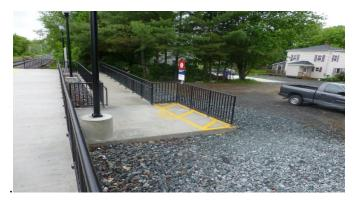
Figure 3-2. Picture Showing A Ramp Leading from the Backside of a Platform to an Emergency Egress Area; The Landing at the Bottom has an Open Side with an Approximately 9- to 12-Inch Drop Off to a Rocky Surface. A parking lot with a truck parked in it is visible in the picture. Source: USDOT
