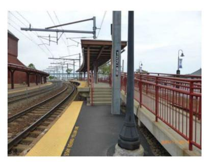
Figure 5-4. Platform with an 8-Degree Curve. Source: USDOT
