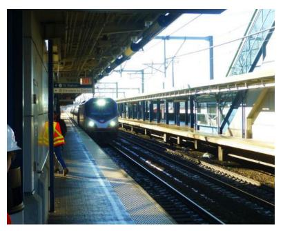
Figure 5-2 shows a platform with level-entry boarding for passenger-only tracks.
