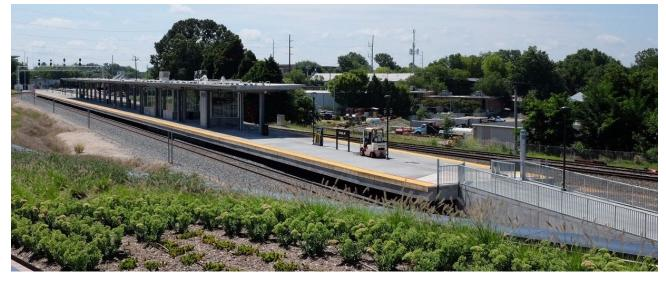
Figure 6-8. Level-Entry Boarding Island Platform with Vertical Access. Source: USDOT
